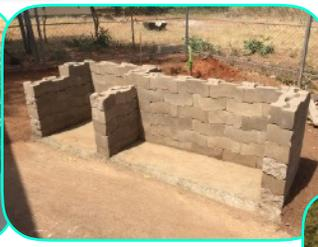
Bill has taken up the challenge to build a barbecue/smoker combination. Once the foundation was poured, Sammy laid the first course of these interlocking blocks. The blocks don't use any mortar, but with their design are very stable. In fact Bill is not a fan at all. He is constantly saying "these blocks give no grace". If they are not put together exactly they will not go together at all.
