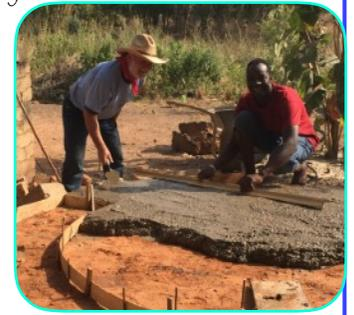
We pour an inner floor of concrete and then lay the remaining block wall up two feet above the floor. Once the wall is complete we dig down beside the wall and construct the nest box below floor level. Then we install the cement tunnel blocks from the nest box to the floor surface. For the roofing, we use vertical posts from local trees, in this case Teak, and the roof is local grass that is thatched.
